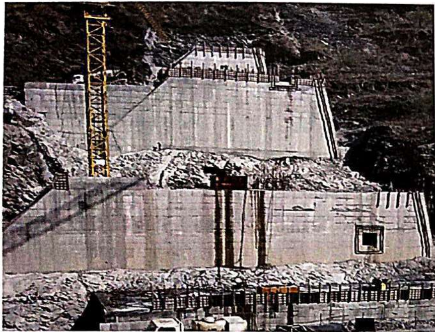
Vyasi Hydro Electric Project – dehradun Contractor : Gammon.
